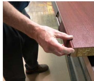
Step 4: Beginning at the top end, flex the vinyl edge and apply pressure to start engagement of the return leg of the vinyl edge into the door kerf. From this end, work down the length of the door engaging the return leg of the vinyl edge into the door kerf until the entire edge is engaged. Reattach any hardware removed in step 1.
