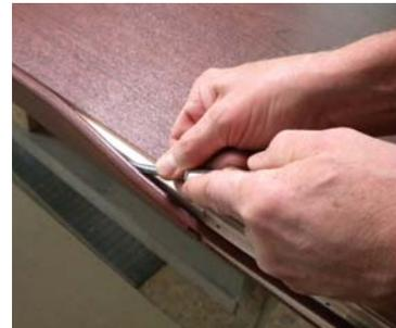
Step 3: Begin attachment of the replacement edge by engaging the return leg of the narrow face into the door kerf. (Note: the replacement vinyl cladding is provided with tape in both edges of the profile. This tape insures proper fit and aids in the impact resistance of the edge and should not to be removed.) To insure proper position, align the vinyl edge to the top end of the door before finishing the installation.
